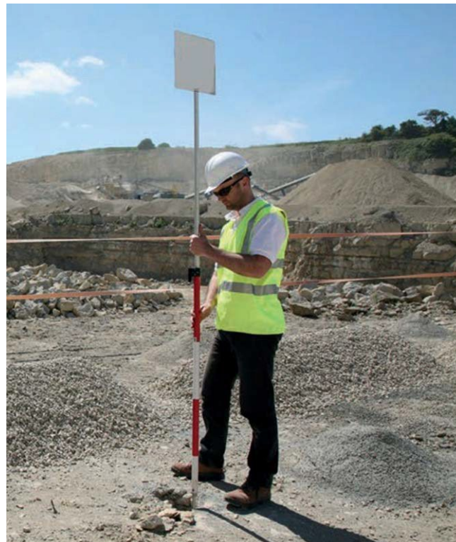
Figure 41 Target on survey pole being used to position a hole collar
